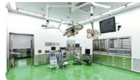
Operating theatre with positive pressure ventilation
