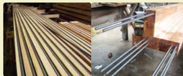
Grooves are added to timber lamellas and then set the steel bars into the timber using an epoxy resin. The rest of the manufacturing process is the same as when producing normal glulam timber.
