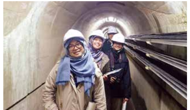
Monitoring tunnel inside the dam.
